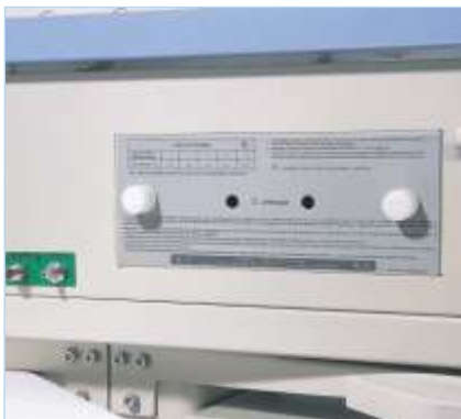
Microfiltered Inlet for O 2 and Air
