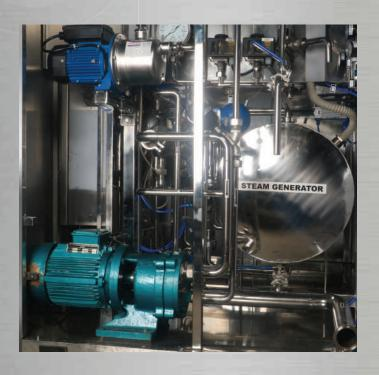
Electrically heated Steam Generator that can self generate steam. This means your sterilizer is independent and can rapidly start the minute you want to sterilize a load.
